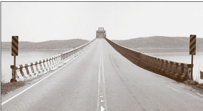
This is how the bridge used to look crossing toward the east. Many broken side mirrors happened because of its narrow lanes.
